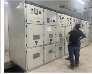
▶ 电气柜调试 Electrical cabinet debugging
